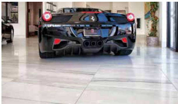
Fig 1. Installations subjected to heavy loads like automobile dealerships should use a tile assembly with a performance service rating of at least Heavy, which means the tested assembly has passed at a minimum cycles 1 through 12 of the Robinson Floor Test. Photo courtesy of Crossville, Inc.
