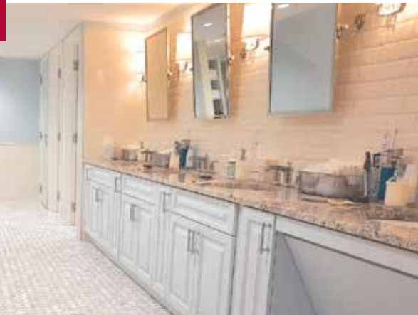
Women's Locker/Toilet Room – Custom Fabricated 1x2 Calacatta Marble Mosaic Basketweave Pattern Floor Tile & 4x8 Sonoma Wall Tile
